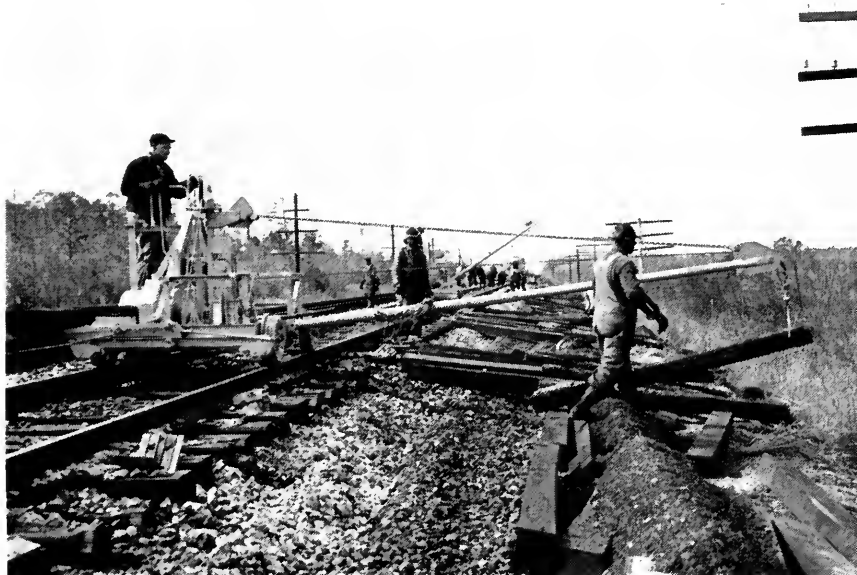
Tie puller and inserter.
